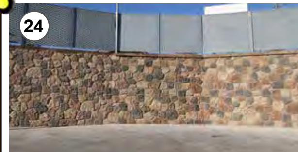
24 - Lavoro ultimato 24 - Completed work
